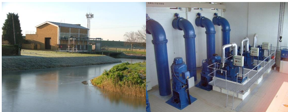
Figures 5-10 and 5-11: Cross Guns Pumping Station inside (left) and outside (right).
